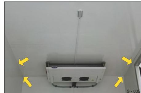
Fig. 20 Bonding the walls above
