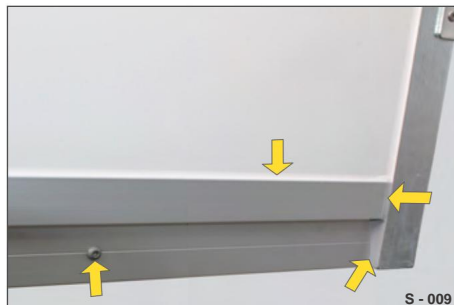
Fig. 9 Bottom chord profiles corner rear side
